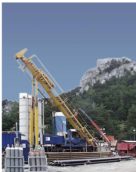
Directional drilling at LTF Avrieux
