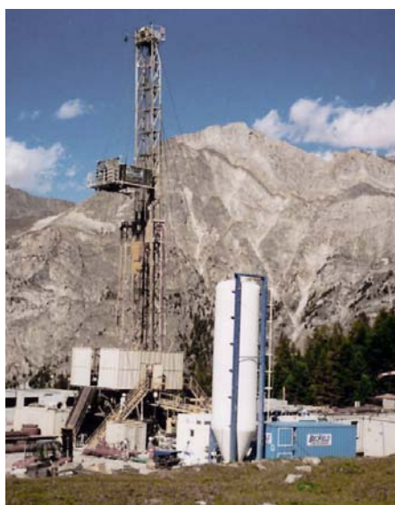
Directional drilling at LTF Etache
